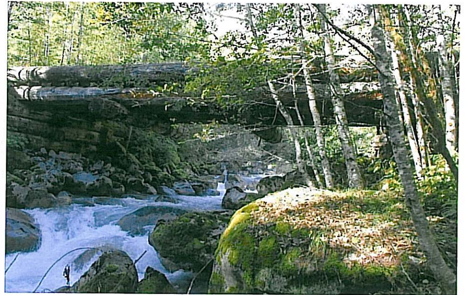
CK-2232 From downstream span 2
