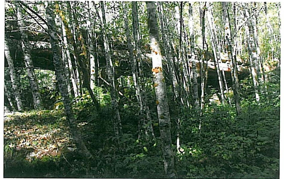
CK-2232 From downstream span 1
