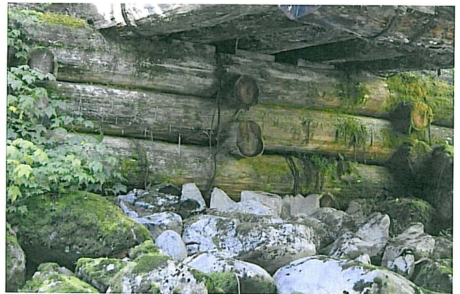
CK-2232 Right abutment
